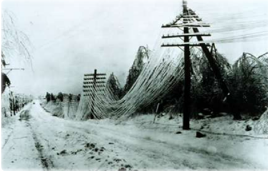
Fig. 1: Electric wires covered by ice
